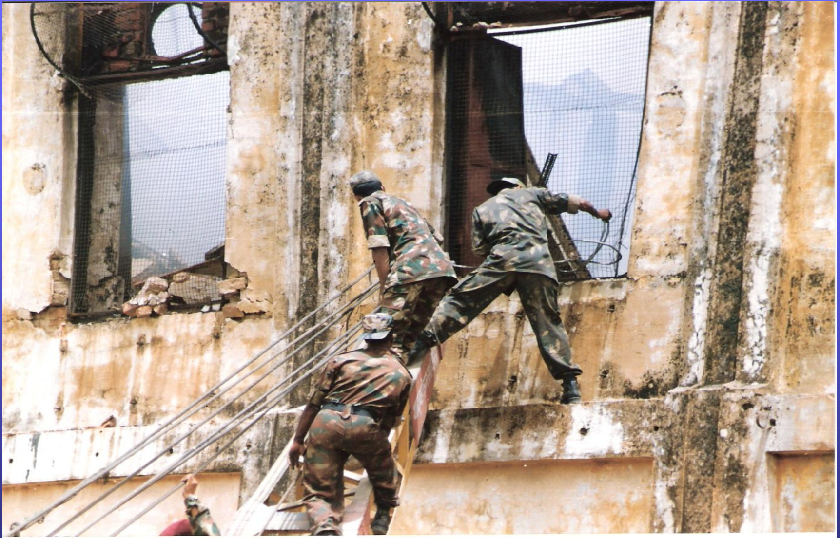
View of window fitted with wire mesh
